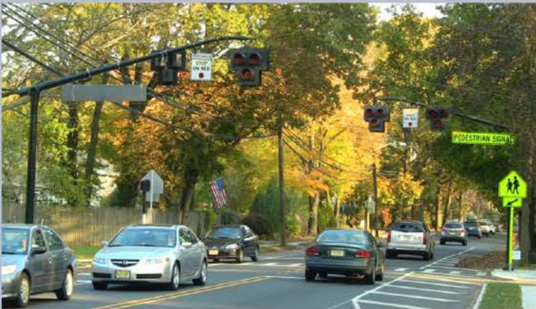
Pedestrian Activated HAWK Signal
